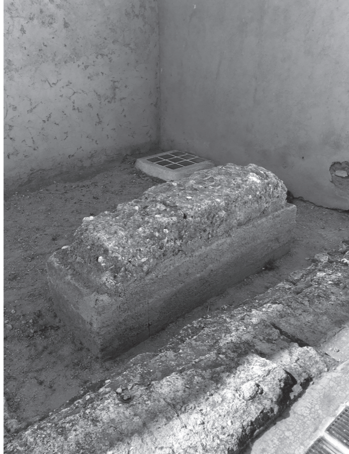
CB-F10-6: Demolished Stone at El Bad Palace, Marrakesh, constructed 1518.
